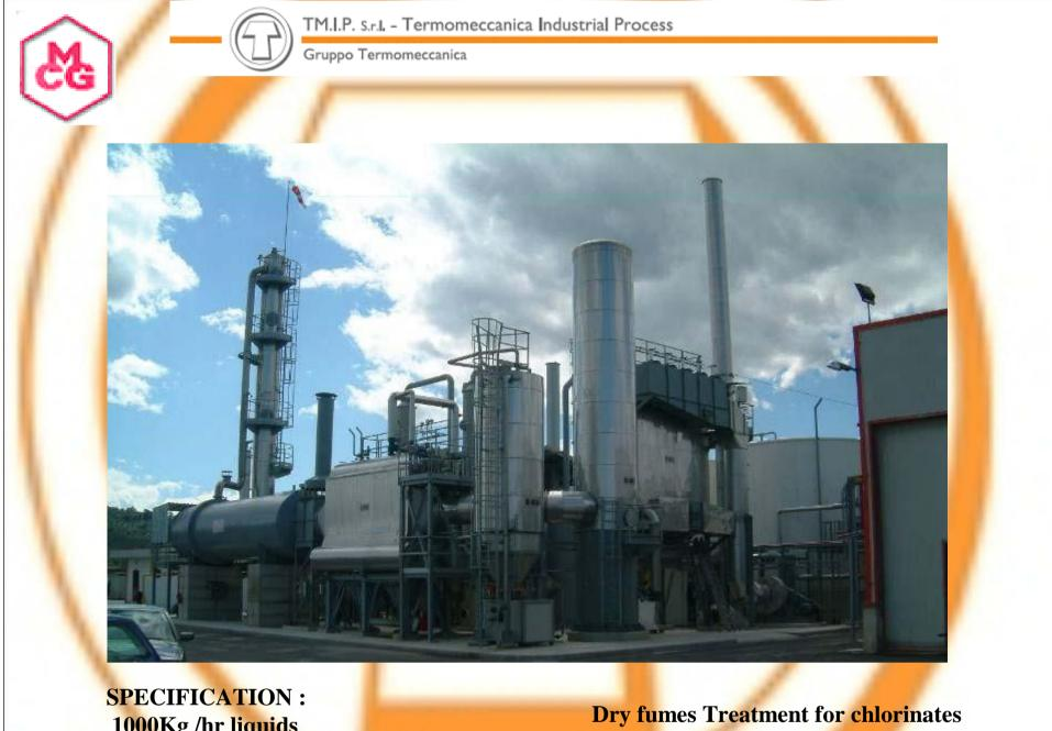
1000Kg /hr liquids 2.000 Nm<sup>3</sup>/hr solvent polluted air Dry fumes Treatment for chlorinates Heat recovery: 5.000 kg/hr of steam
